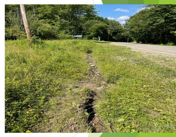
Pictured above is an erosion path that can be seen along the north bank of Moore road. This project will incorporate check dams and native plantings to reduce stormwater velocity and prevent erosion.
