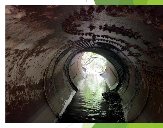
Pictured above is a view inside the existing aged culvert. A seam has separated allowing sediment infiltration (bottom right).
