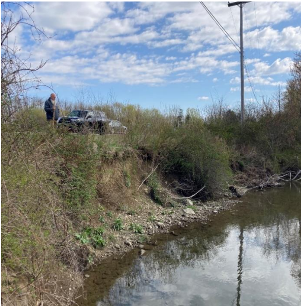
Pictured above is the Stow Road bend of Ball Creek prior to construction.
