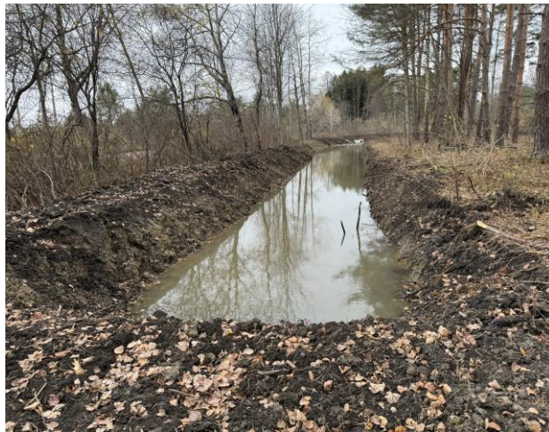
Photo of the north stormwater channel during construction.
