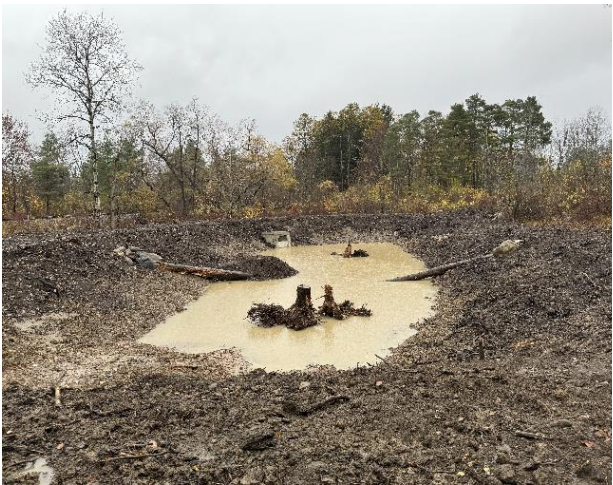
Photo of the east wetland during construction.
