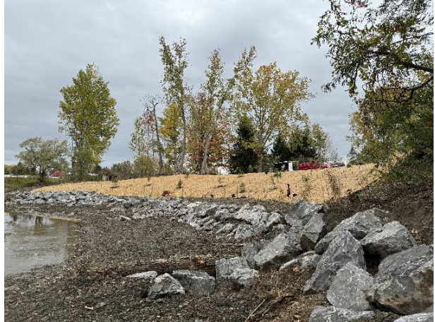
Photo 2. Ball Creek 10/11/23 after construction.
