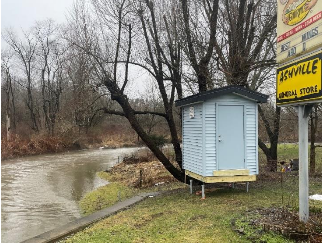
Pictured above is a stream station under construction along Goose Creek.
